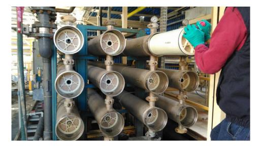
Pressure vessels in a reverse osmosis unit in Turkey are loaded with Lewabrane RO membrane elements from LANXESS. Photo: Burkut
